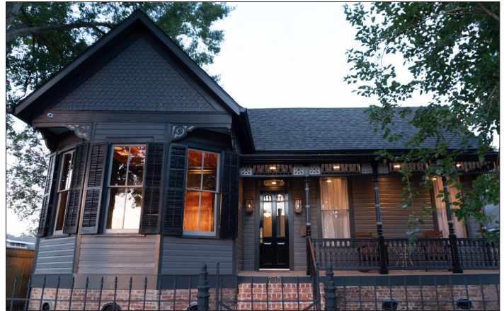
700 Monroe St. after restoration
