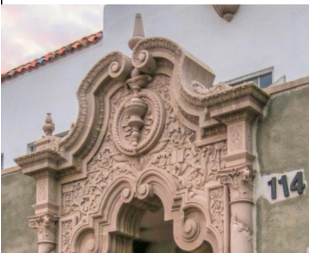
Carpentry Tools surround the door of the Marcus Feingold Mechanical & Arts Building.
